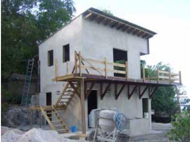
Construction of the new dive facilities.
